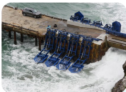
Figure 2 : Dispositif Eco Wave Power point absorber
